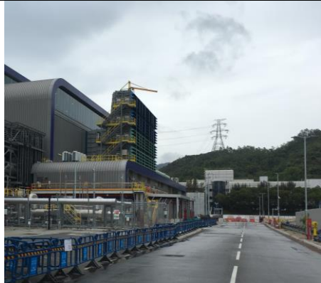
Reinstatement of road after the construction of CCGT Unit No.1
